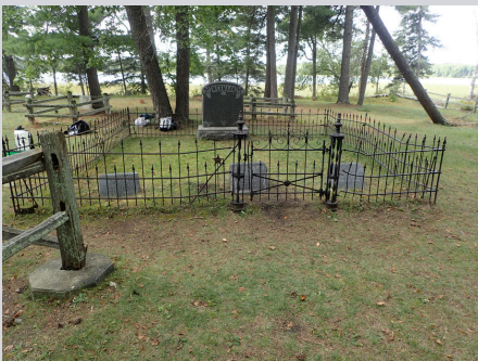
A photo of the monument and fence after cleaning.
