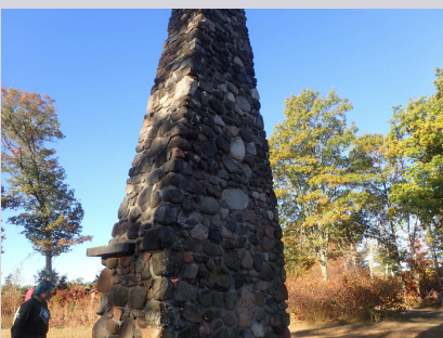
The chimney after repointing.
