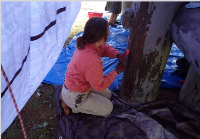
Corpsmember prepping log for repair.
