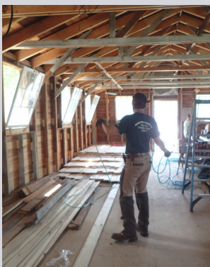
Corpsmember prepping floor to be replaced.
