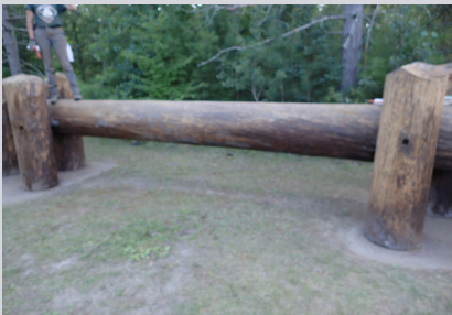
An after photo of the log restoration work performed by Corpsmembers.
