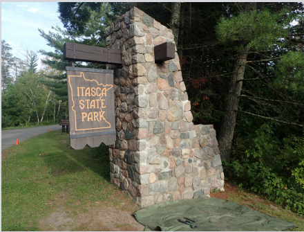
A photo of the Itasca State Park East Entrance before repointing.
