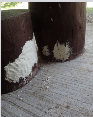
A during photo of the pillars.
