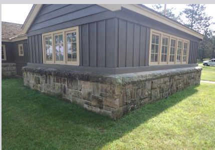
A before photo of uncleaned masonry.
