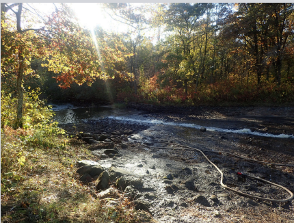
The spillway after cleaning.
