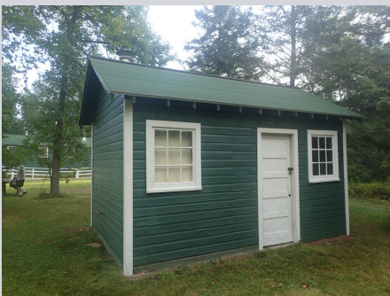
A photo of the repainted pumphouse.
