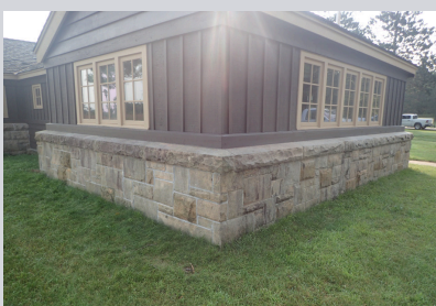
After photo of cleaned masonry.
