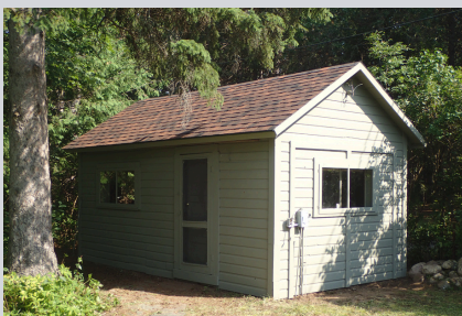
Sigurd Olson's writing shack after siding and shingle replacements.
