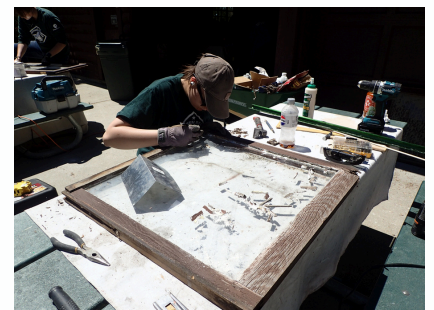
Corpsmember removing glazing from historic window.
