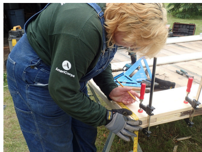
Corpsmember repairing the oil shed door.
