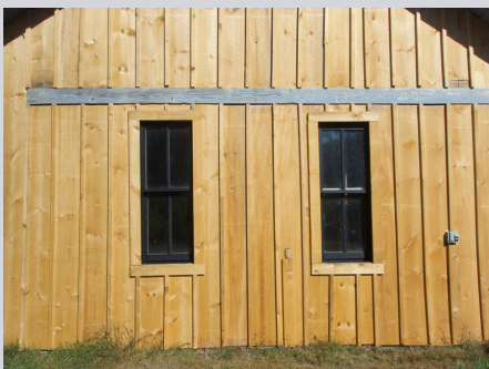
A photo of the window after repair.
