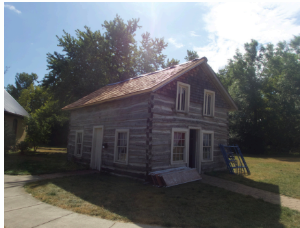
A photo of the roof after repair.
