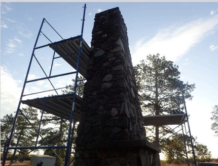
The chimney before repointing.
