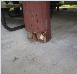
A before photos of the pillars.
