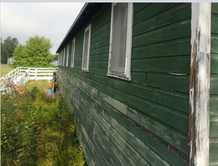
Corpsmember painting and scraping bathhouse.
