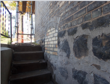
Restored and cleaned brick.
