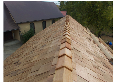
A photo of the newly installed cedar shingles.
