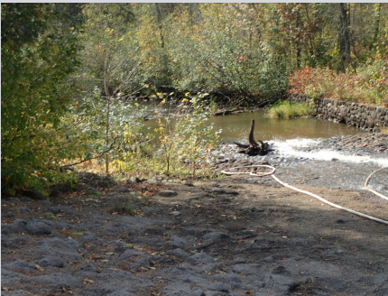
The spillway before cleaning.
